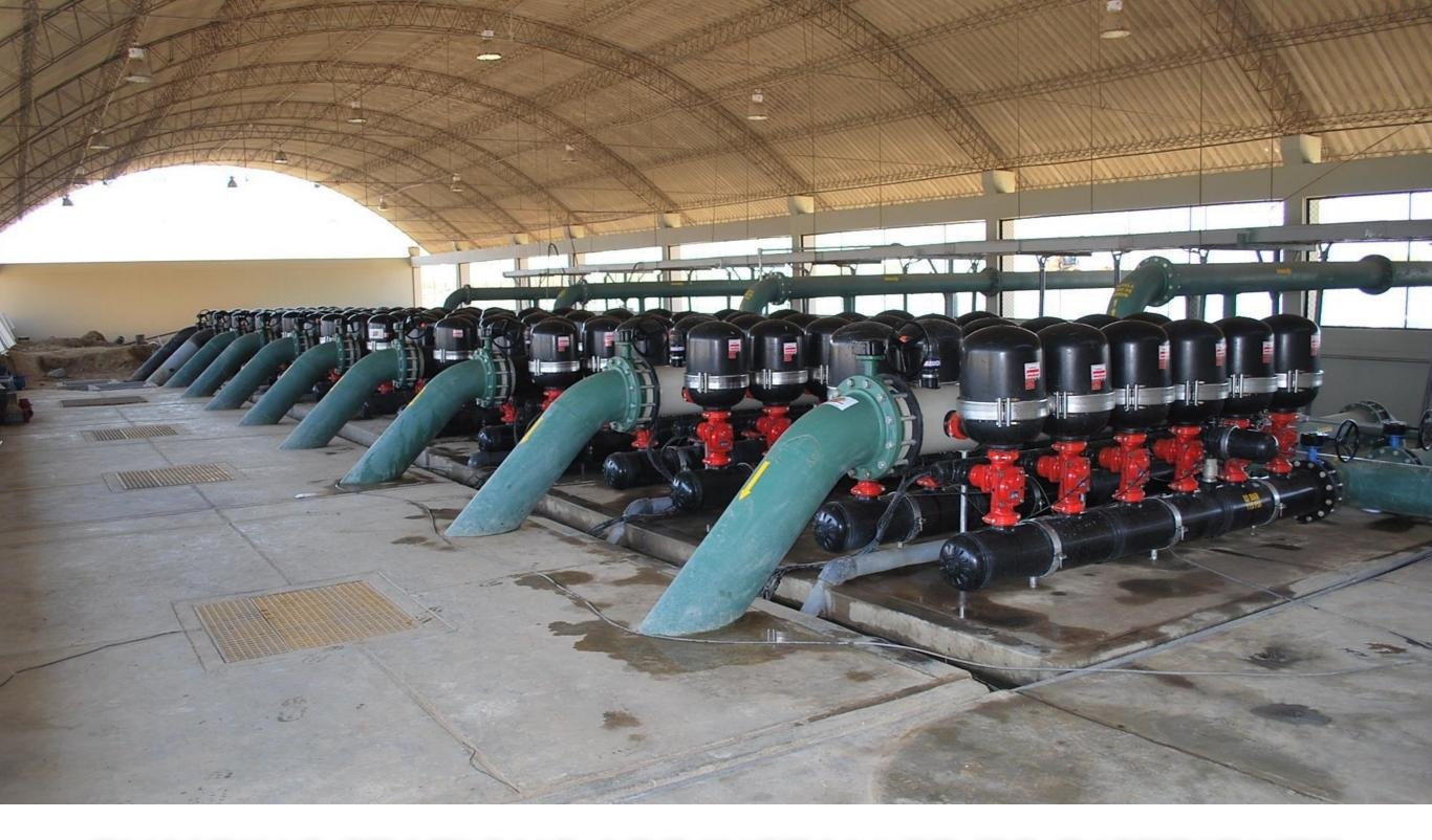
PUMPING STATIONS ARE INSTALLED TO DISTRIBUTE WATER AT A RATE OF NEARLY 12,000 M3/HA PER YEAR
